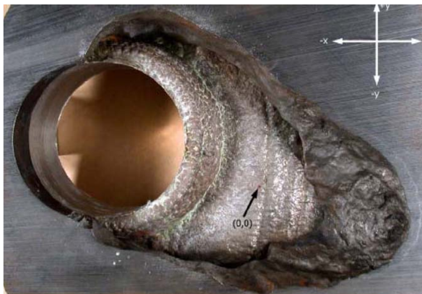
Figure 4 - Davis-Bessie Reactor Vessel Head Cavity (NRC Website)
